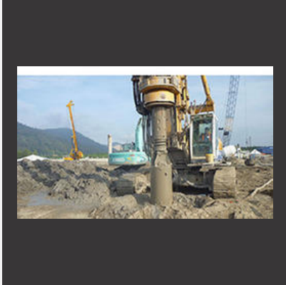
Pile Construction Service
