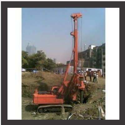
Hydraulic Rotary Piling Service
