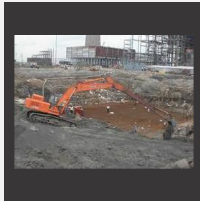
Excavation/ Rock Blasting / Mining Contracting Services
