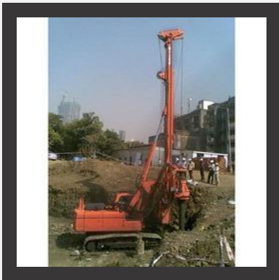
Hydraulic Rotary Piling Service
