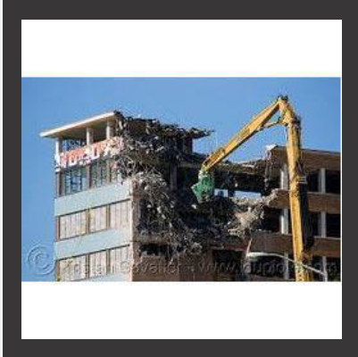
Building Demolition Services
