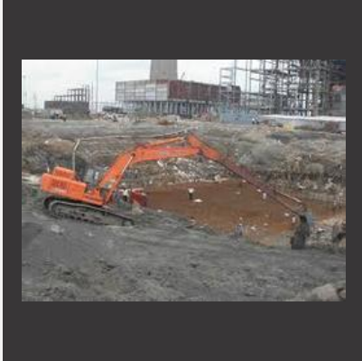
Excavation Contracting Services
