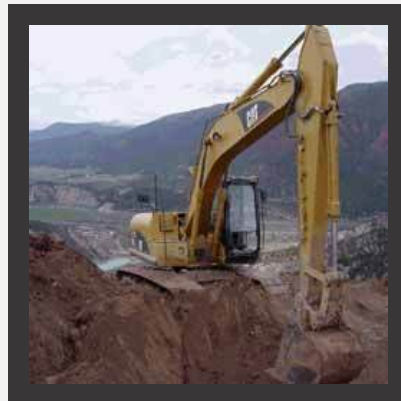
Rock Excavation Services
