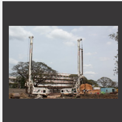
Bored Cast In Situ Piles Services
