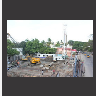
Pile Foundation Contractor Service
