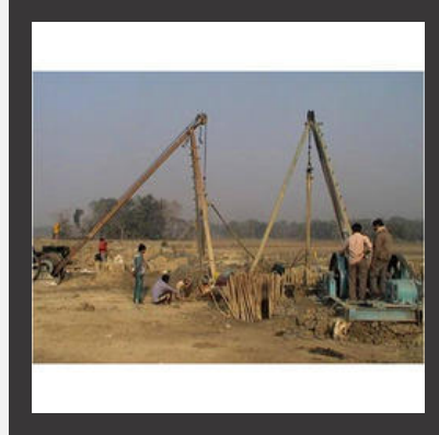
Pile Foundation Service
