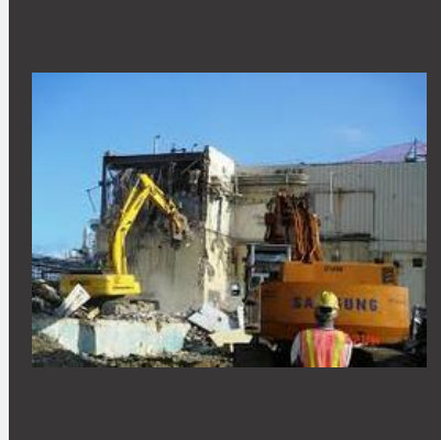
Industrial Demolition Services
