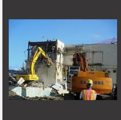
Industrial Demolition Services
