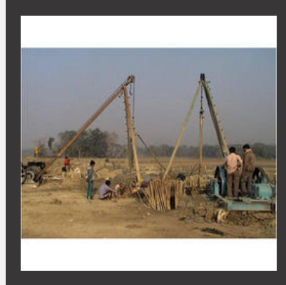
Pile Foundation Service
